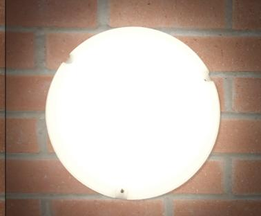
**STEP 6**Secure diffuser in place
